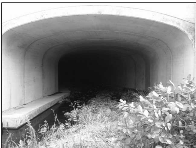
Example of bottomless culvert; note natural bottom material remains
