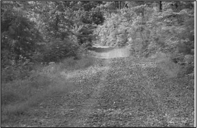
Example of broad-based dips. Murray County, Georgia Photo: Courtesy of Limestone Valley RC&D Council
