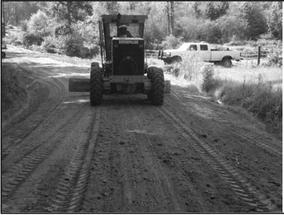
Re-shaping crown step 4: final shaping.
