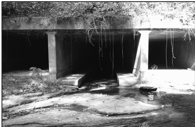
Example of fish passage culvert. Pickens County, Georgia
