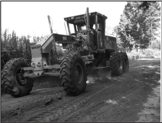
Re-shaping crown step 2: re-distributing road surface.
