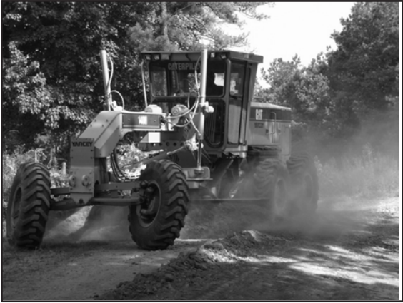
Re-shaping crown step 1: cutting road surface.
