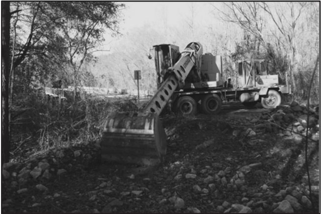
Removal of stored sediment after 3 full. Lamar County, Georgia Photo: Courtesy of Two Rivers RC&D Council
