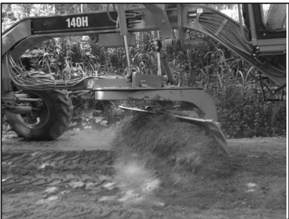
Re-shaping crown step 3: re-mixing road surface.
