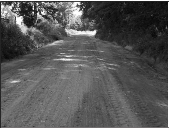
Re-shaping crown: completed.
