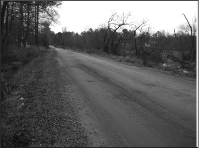
Unpaved road adjacent to wetland (right shoulder); note vegetated shoulder, banks and ditch to trap sediment. Lamar County, Georgia Photo: Courtesy of Two Rivers RC&D Council
